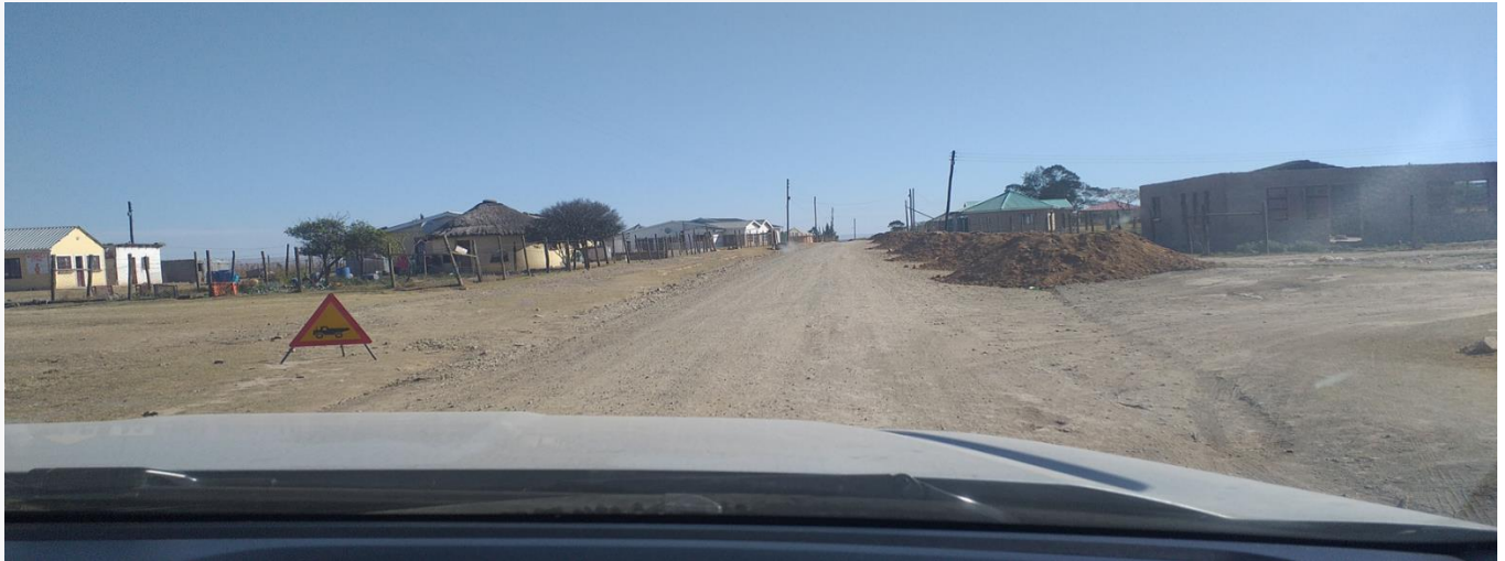
Surface Street (Pothole Patching in ward 13, North crest, Jizana Street.
