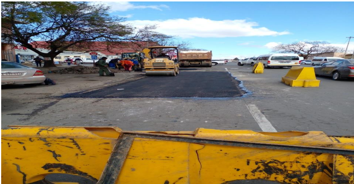
Surface street (Pothole Patching in ward 13, North crest, Jizana street.
