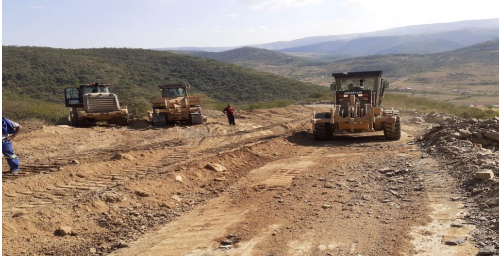
Regravelling of road in ward 21 Thamsana
